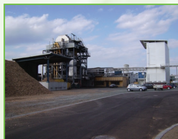
The CHP Güssing and the BioSNG plant nearby
