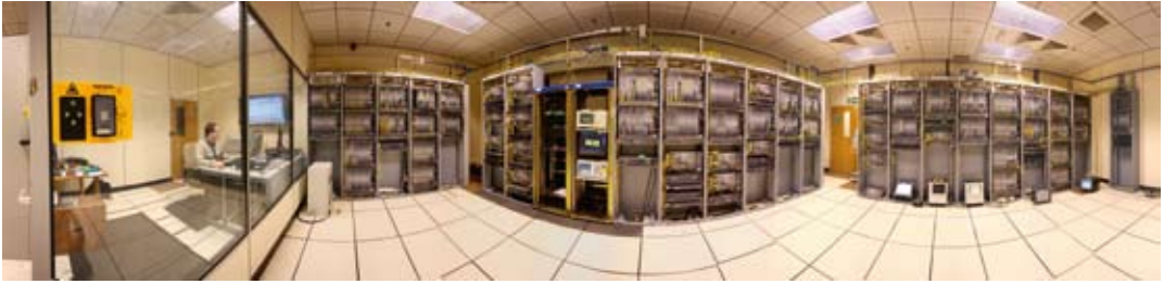
Fig. 4.1.17 System test environment © Ericsson
