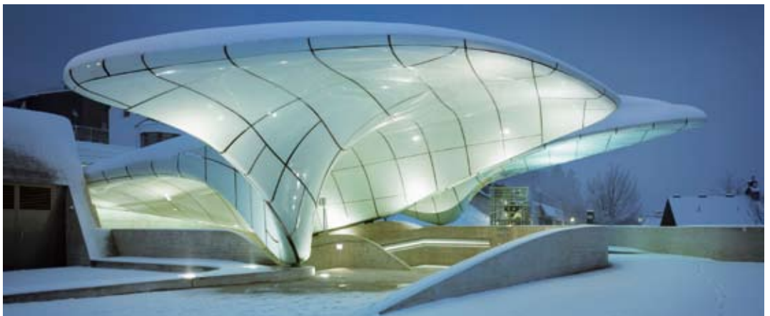
Fig.4.4.17 LED solutions contribute to impressive modern architecture © Zumtobel
