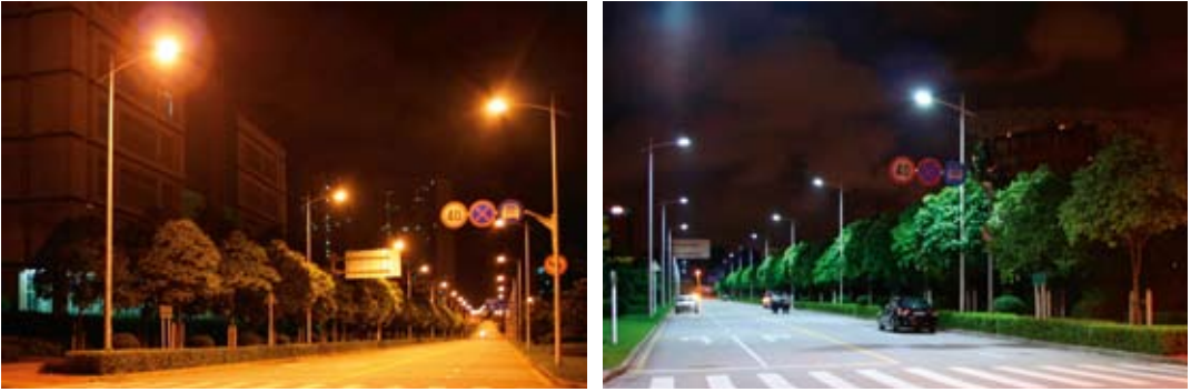
Fig. 4.4.21 A street lit by high-pressure sodium lamps (left) after conversion to LED lighting (right) © OSRAM Opto Semiconductors
