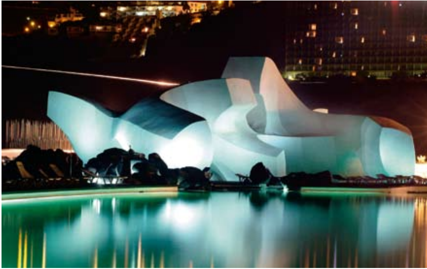
Fig. 4.4.2 LED floodlight illuminates the Lagoa Martiñez complex in Puerto de la Cruz, Tenerife © Philips
