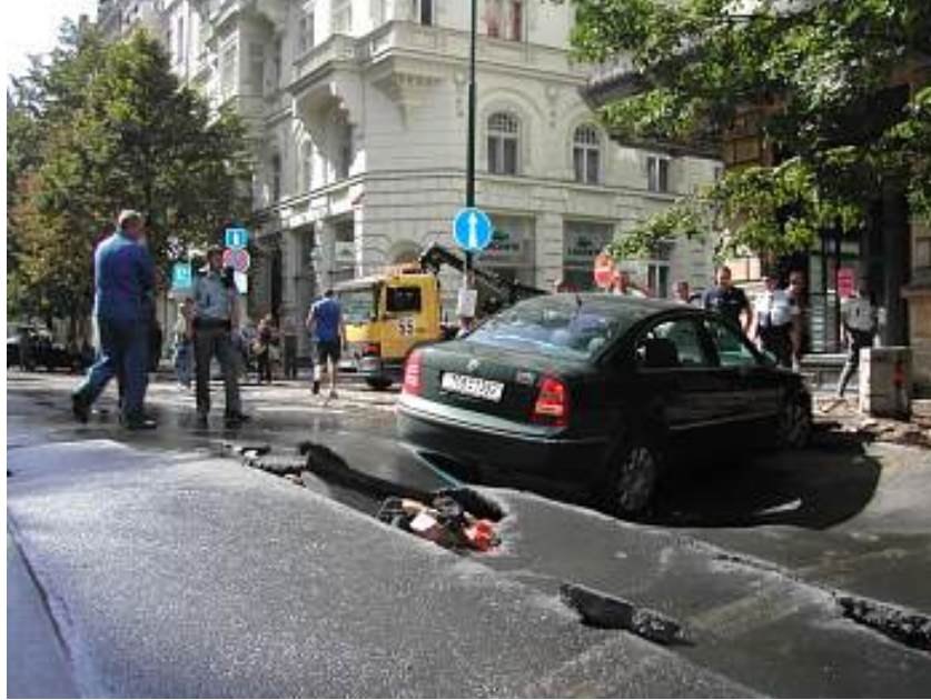
Burst water main, Prague
