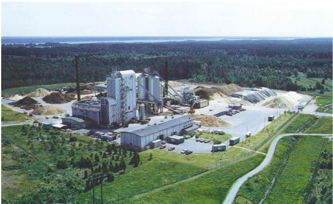
Värnamo gasification plant – earlier used for electricity production, now rebuilt to produce synthesis gas for transport fuels.
