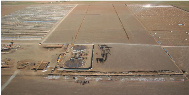
Troughs (aerial view of Andasol plant under construction)
