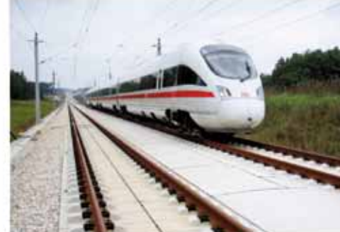
SAS Threadbar-System on the new ICE high speed railway
